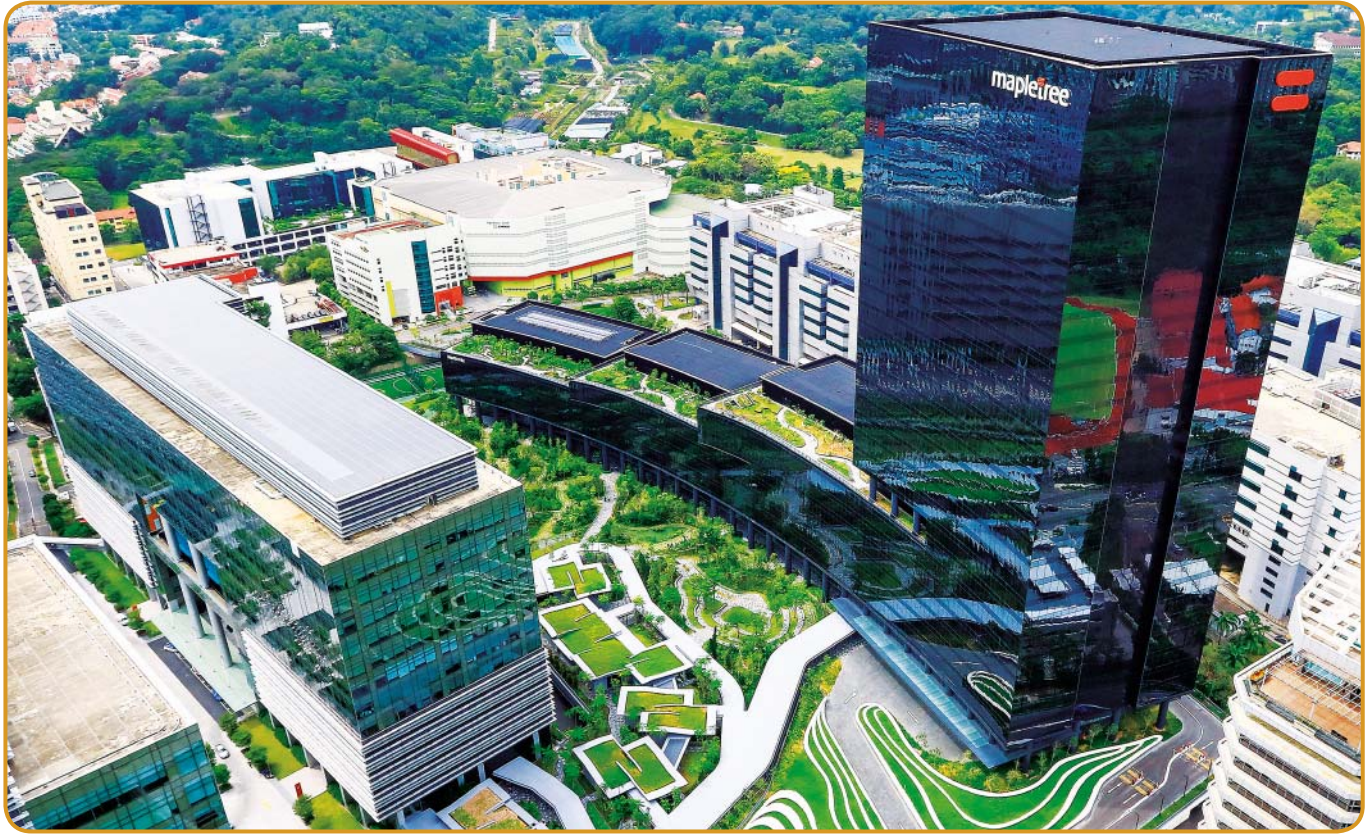
Mapletree Business City (MBC) is the Group's flagship development in Singapore and has attained several notable awards for its sustainable features which include an efficient chiller plant and green roofs amongst others
